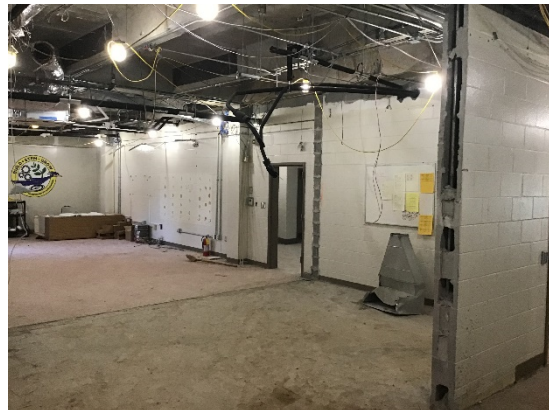
Hallway CMU Wall Demolition
