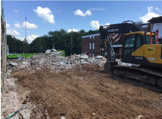
Building Slab Removal
